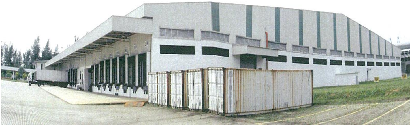
EXTERNAL VIEW OF WAREHOUSE
